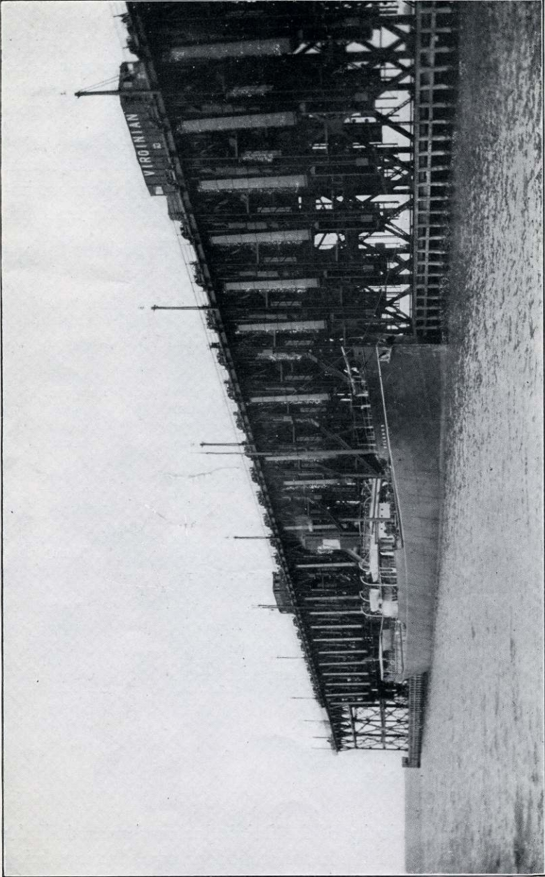
The out-shore end of coal pier showing adjustable chutes and two conveyor cars. The unloading is done by the Company at the expense of the shipper or consignee.
