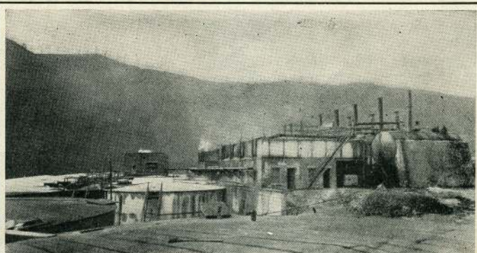
Oil tanks and refinery, Kanawha Valley
