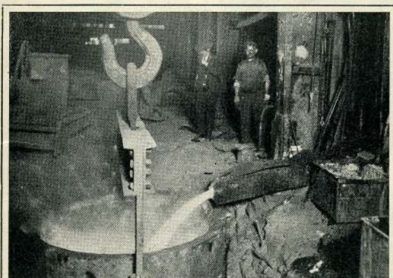
Pouring molten metal in steel plant, Wheeling
