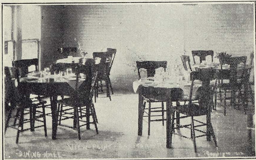
DINING ROOM VIEW POINT SANITORIUM
