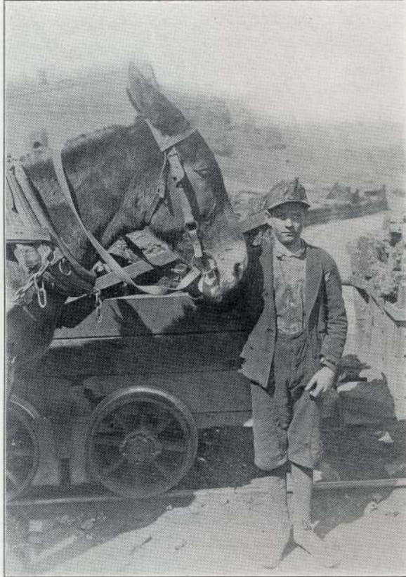
Photo, October, 1908, by Lewis W. Hine.
