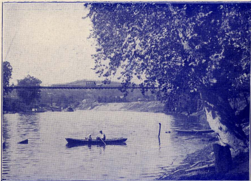
OLD SUSPENSION BRIDGE ACROSS ELK RIVER—FELL DEC. 15, 1904.
