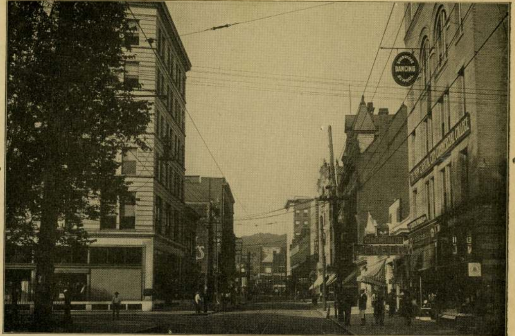
CAPITOL STREET, LOOKING SOUTH FROM STATE
