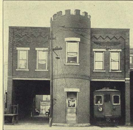
PARKERSBURG FREIGHT OFFICE AND STATION
