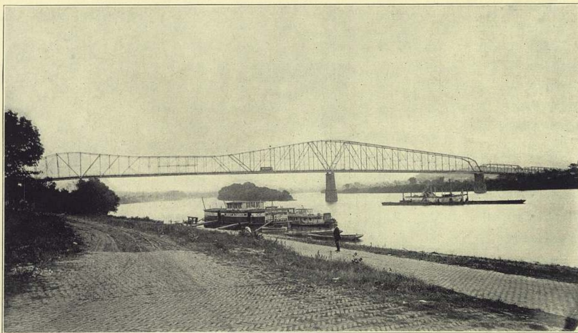
A VIEW OF THE OHIO RIVER BRIDGE
