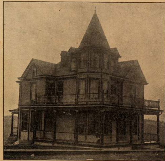
Residence of D. B. PURINTON, LL. D., President of the W. V. U. On lot No. 18, block 54
