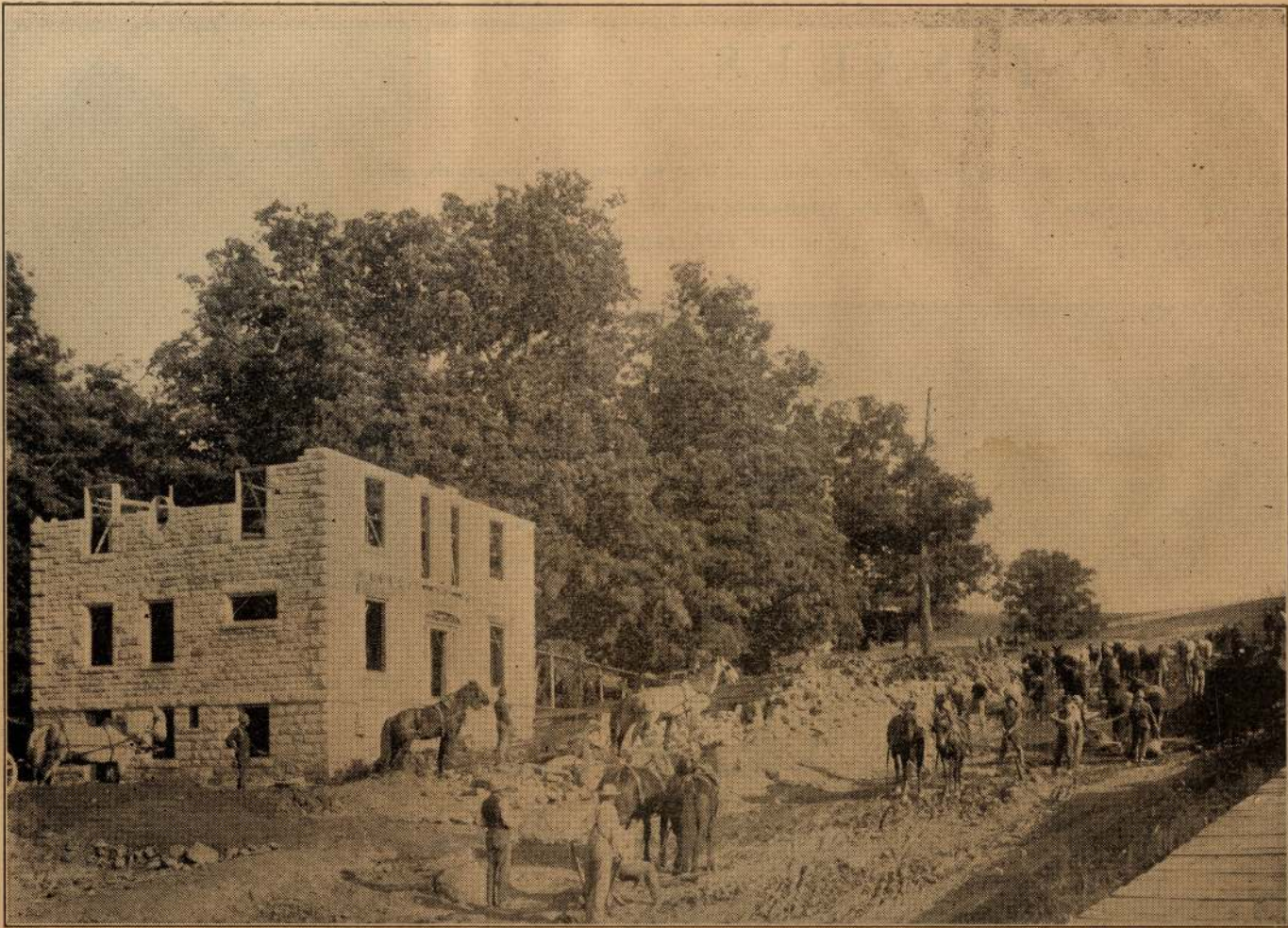
A BUSY SCENE. GRADING GRAND STREET, SOUTH PARK
